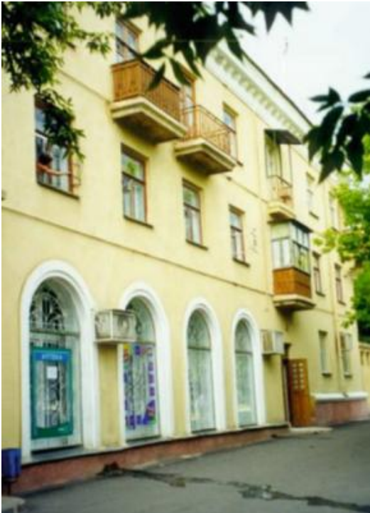
Figure 3. Residential building - precast blocks made from alkali hydroxide-activated slag, Mariupol, Ukraine [17]
