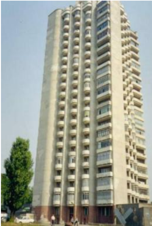
Figure 2. High-rise building made from alkali carbonate-activated slag, Lipetsk, Russia [17]
