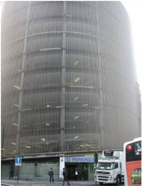
Figure 5. The “Parking 58”, Brussels, Belgium – parts of the first six floors are built from Purdociment [17]
