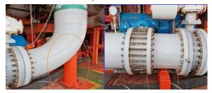
The job started by checking the suction strainer, but there was no strainer, strainer was removed a long time ago Currently there is no suction strainer at the suction line. The ammeter was calibrated due to showing abnormal readings in comparison with other motors and accordance with the readings of the control room.
